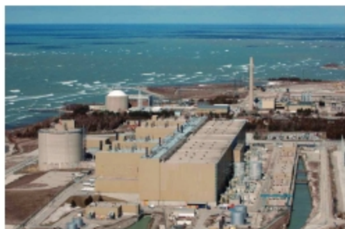
Bruce Power Generating Station, Kanada
